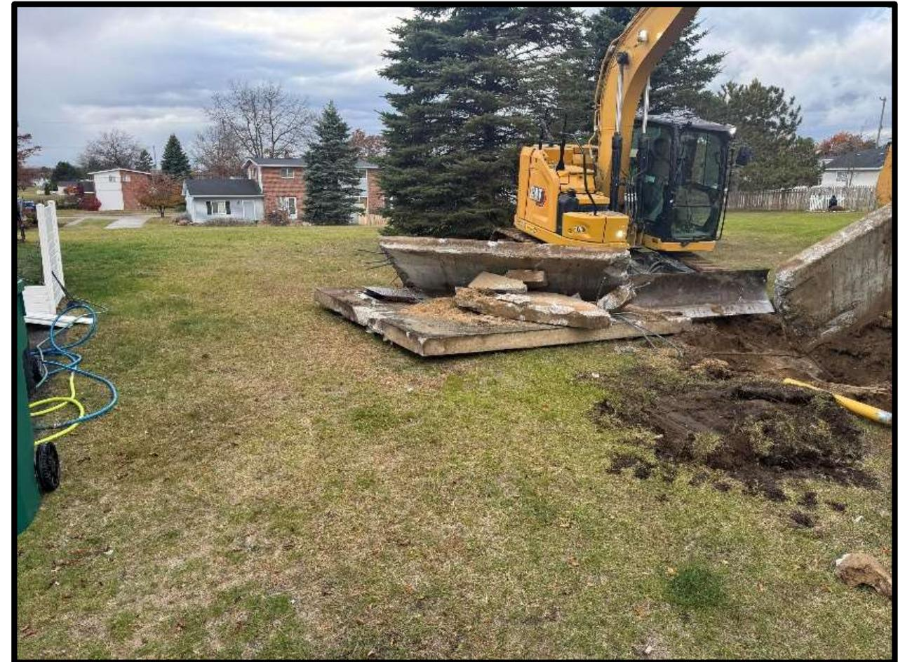
Concrete debris and associated materials were removed and transported for off-site disposal
